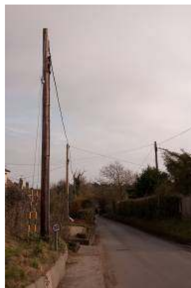
Residents want cables put underground
