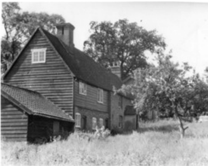
Mill Cottages, empty in 1961, prior to refurbishment
