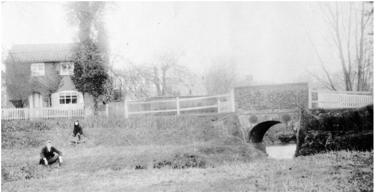
Bridge Cottage viewed from the Cricket Meadow; the bridge was replaced in 1894
