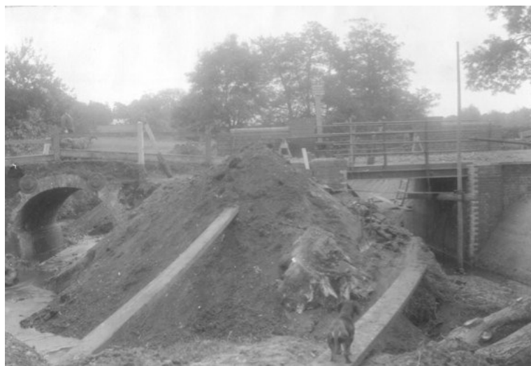
The new bridge, right, nears completion while the old bridge awaits demolition. Looking east from the Cricket Meadow, Hill House (then colour-washed) is just visible in the background
