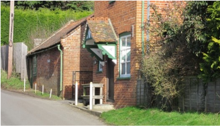
The brick shed, left, was used by Amos both as a store and an outlet for his produce. On his retirement in 1887 the purpose built shop, centre, was set up on an empty piece of land, a prominent corner site adjoining Copyhold
